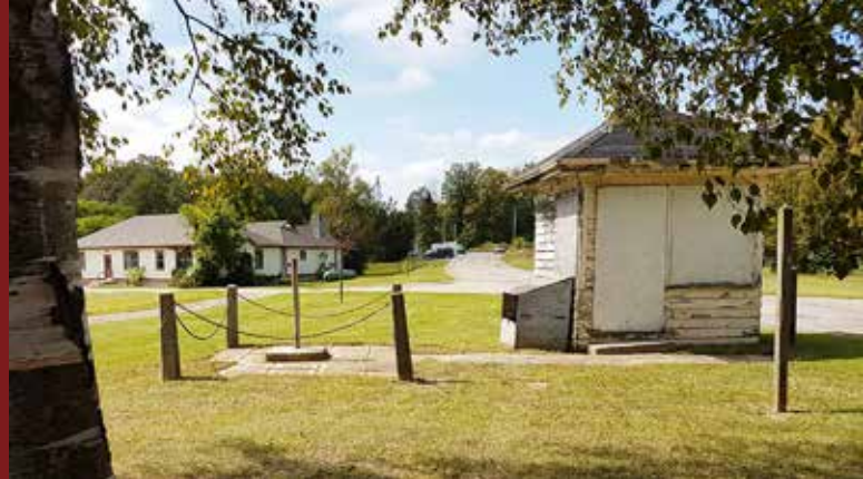
A view of the historic gatehouse that will be restored in 2019.
